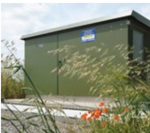
Medium Voltage electricity
