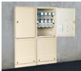
Low voltage electricity
