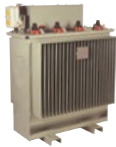
Auxiliary supply transformer
