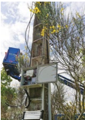
Pole-mounted substation - data measurement and communication system
