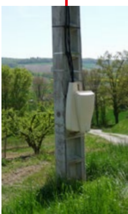
TRAFFIX Pole-mounted LV switchboard
