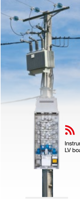
Self-protected pole mounted transformer
